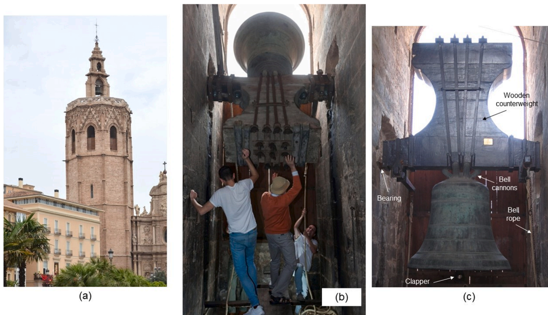
Fig. 1. (a)- El Micalet bell tower. (b)- Bell ringers ringing the bell manually (c)- El Jaume bell.
