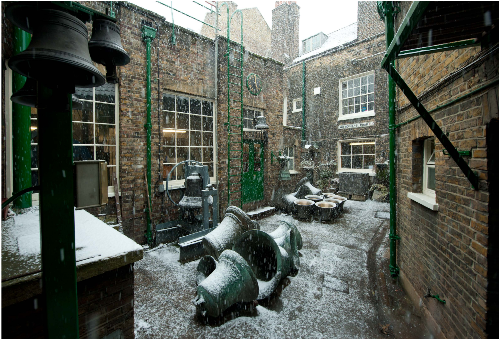
The internal yard or area from the southeast in 2011 (photograph by Derek Kendall, © Historic England Archive)
