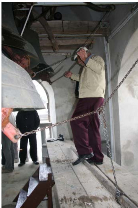
Figure 2: Chiming with levers;
